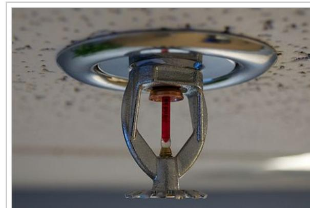
A glass bulb type sprinkler head will spray water into the room if sufficient heat reaches the bulb and causes it to shatter. Sprinkler heads operate individually. Note the red liquid in the glass bulb.
